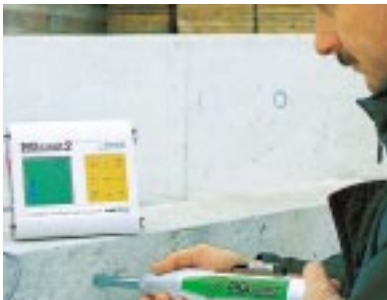
Measuring depth of concrete cover with a Covermeter
